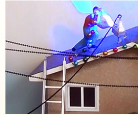
A man attaching seasonal lights on a roof makes contact with a line
