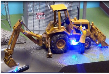
A backhoe contacts an underground line
